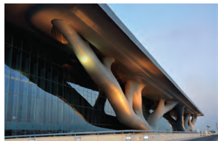
National Convention Centre, Qatar
