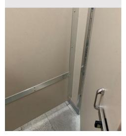
The original HDPE partitions (pictured) required additional hardware to achieve the desired privacy. Evolve achieved the desired panel size without added brackets and its soft-close doors eliminated previous issues with loud hinges.
