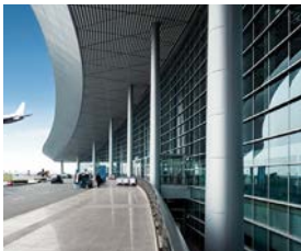
Heavy Traffic Facilities
