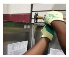
3a. Align the new door with the cabinet and insert the new hinge pin from the top of the cabinet.
