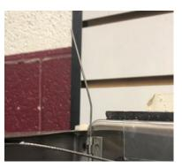
Ensure the newly installed pin is not protruding from the hinge. A hammer or mallet can be used with a file to ensure the hinge is flush.
